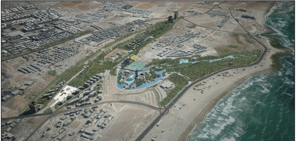
Figure 4.5: A view of the whole project of The New Sindibad project
