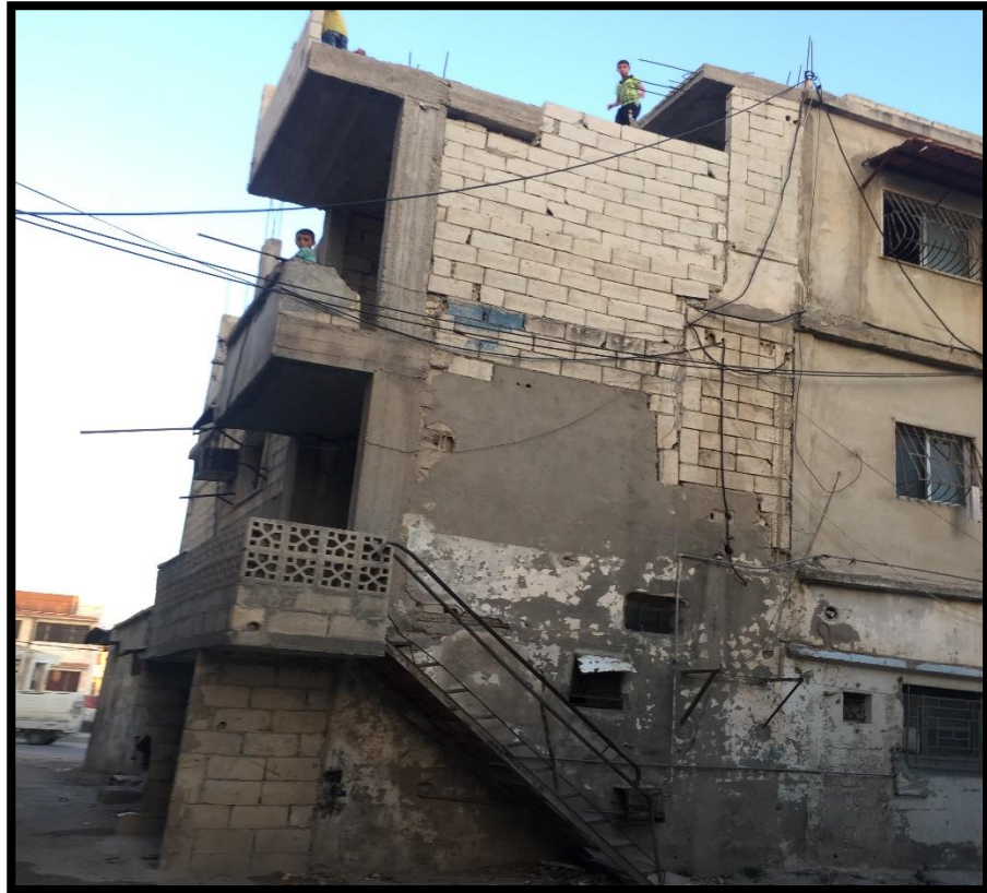
Figure 5.8: Temporal structure with bricks walls in Corniche region
