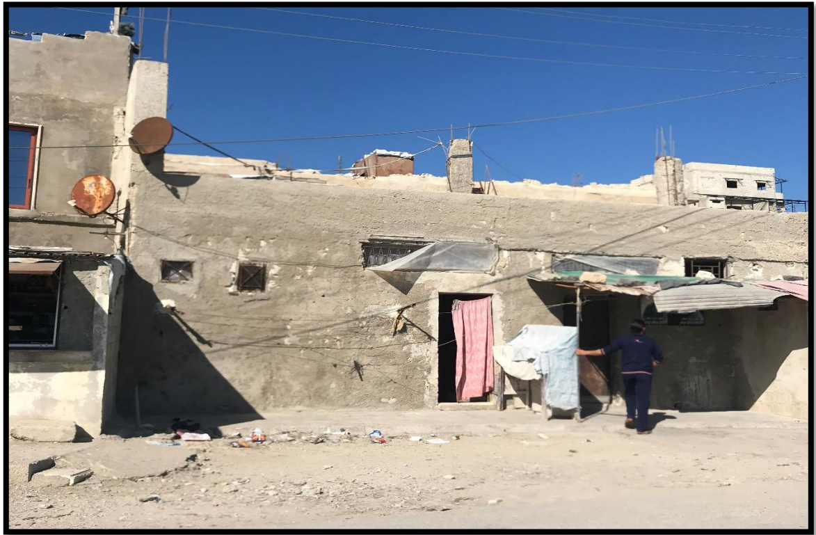
Figure 5.7: “Houses” were built without building plans foundations in Corniche region.
