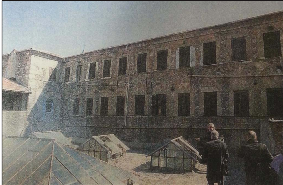
Figure 4.9: Skylights of St. Pierre Han
