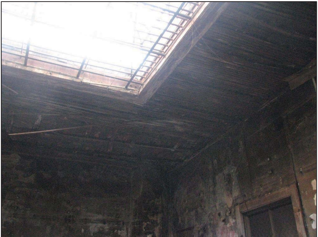
Figure 4.26: Skylights from inside of the han building
