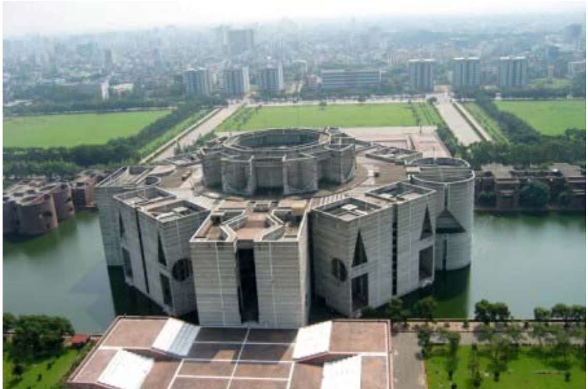
Figure 4.10: Aerial view of the national assembly building
